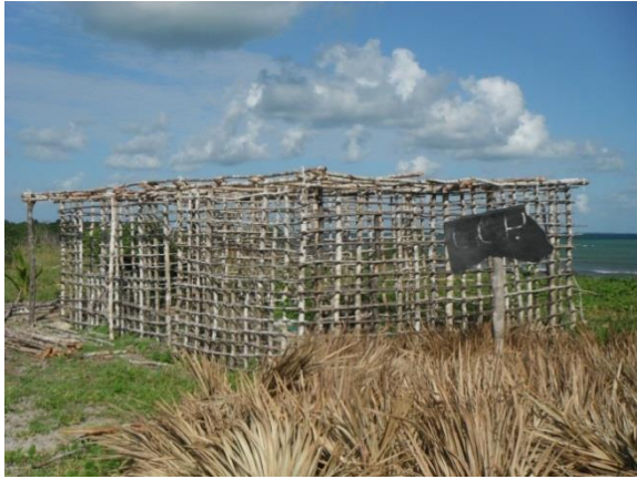
Figure 2. Construction of the CCP office in Quiwie
